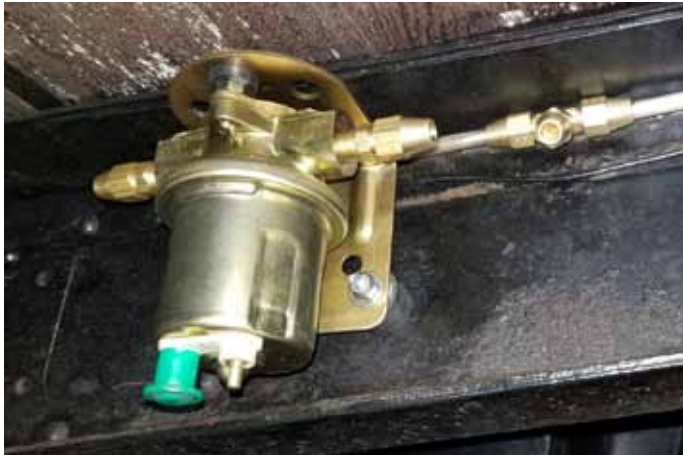
6. First joint is a T-fitting that will feed the electric pump. The main line is routed against the frame behind the electric pump, following the path of the original fuel line.
