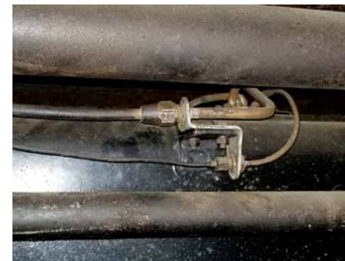
1. Fuel line connection at the fuel tank. You will have something similar on your car. Follow the fuel line forward until you find a suitable place for the electric fuel pump to live. Try to get the electric pump as close to the tank as possible and below the level of the fuel tank outlet so it will self-prime. Smaller line is for the fuel gauge.
