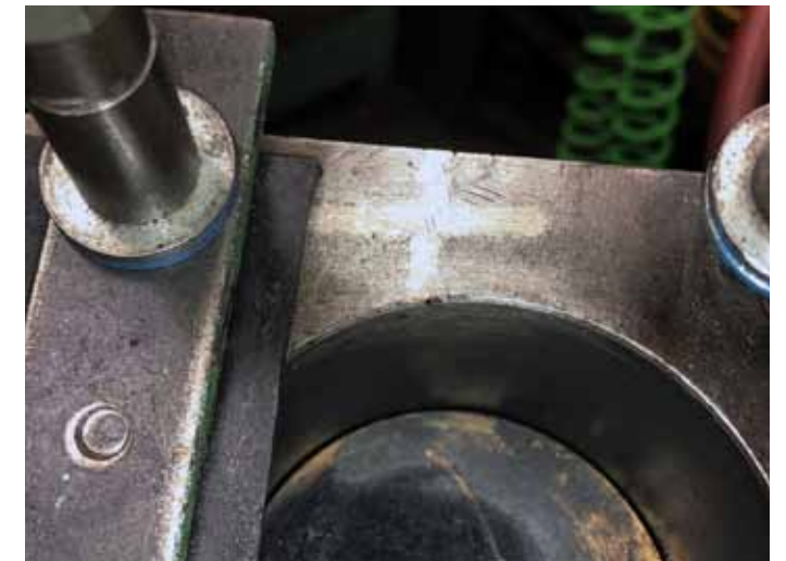
Deck surface crack repaired and machined flat.
