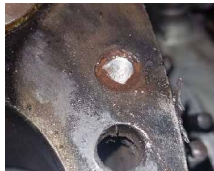
35 out of 58 studs broke off just like this. You can see how corroded and compromised they were.
