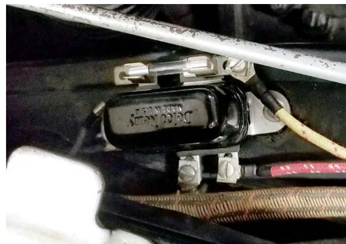
Relay connected [yellow/red = +6V power, red/white = from dash switch, black = ground, white (behind wiring harness bundle) = 6V to fog lights]
